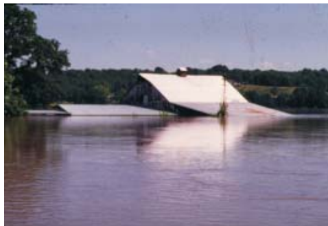
Inundated flood plain and farmstead during the Great Flood of 1993 on the upper Mississippi River.
