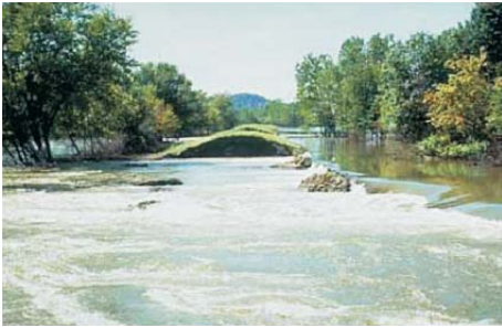
Levee surrounding Clarence Cannon National Wildlife Refuge, Missouri, damaged by the Great Flood of 1993 (Courtesy of U.S. Fish and Wildlife Service)
