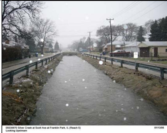
05530670 Silver Creek at Scott Ave at Franklin Park, IL (Reach 5) 01/13/05 Looking Upstream
