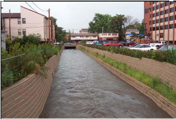
03337100 Boneyard Creek at Lincoln at Urbana, IL Looking Downstream from Gregory St
