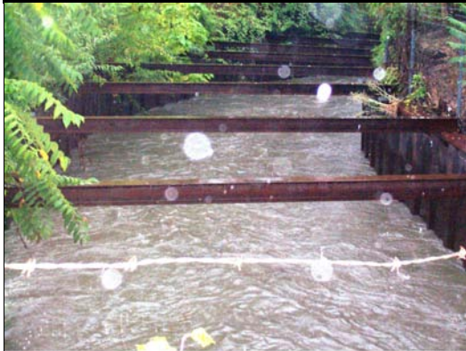
03337250 Boneyard Creek at Race St at Urbana, IL Reach 2 Looking Upstream from Griggs St bridge 08/29/03 n = 0.022 - 0.026
