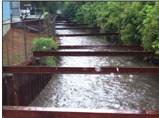
03337250 Boneyard Creek at Race Street at Urbana, IL Reach 2 Upstream of Race St bridge 08/29/03
