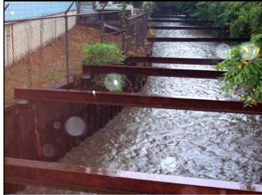
03337250 Boneyard Creek at Race St at Urbana, IL Reach 2 Looking Upstream from Griggs St bridge 08/29/03 n = 0.022 - 0.026
