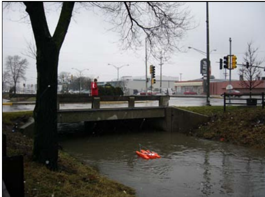
05530690 Silver Creek at 17th Ave at Melrose Park, IL (Reach 2) Looking Upstream at downstream side of Broadway bridge 01/13/06
