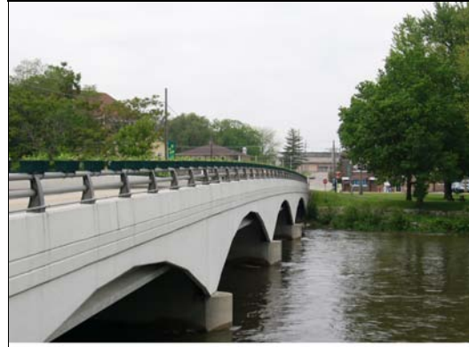
05551540 Fox River at Montgomery, IL Upstream side of bridge
