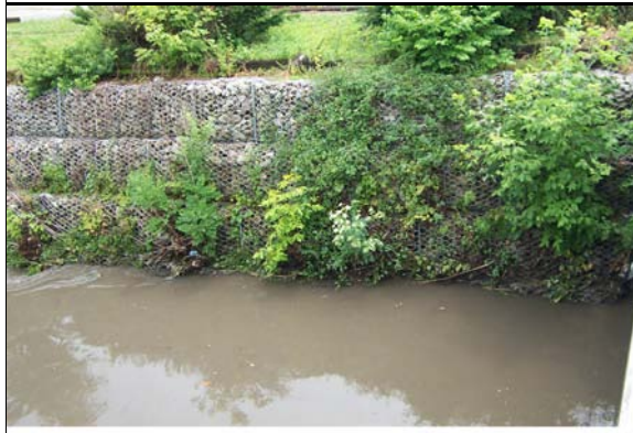
03337250 Boneyard Creek at Race Street at Urbana, IL Reach 1 From Broadway St bridge, looking at right bank gabion boxes 6/10/04
