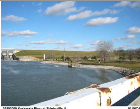
05592000 Kaskaskia River at Shelbyville, IL Looking Upstream from bridge 01/06/04 n = 0.077
