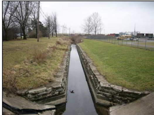
03343200 Embarras Tributary at Champaign, IL Looking downstream from upstream end
