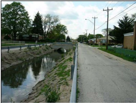
05530670 Silver Creek at Scott Ave at Franklin Park, IL (Reach 5) 05/02/06 From downstream, looking upstream
