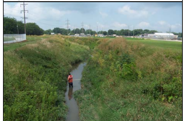
03343800 Kickapoo Creek at Mattoon, IL Looking Upstream from S 9th St bridge 07/21/03
