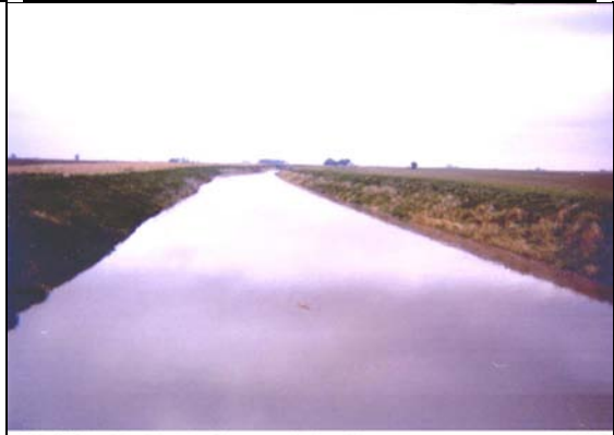
05554000 North Fork Vermilion River near Charlotte, IL Looking Upstream from 3300E 05/15/03 n = 0.023
